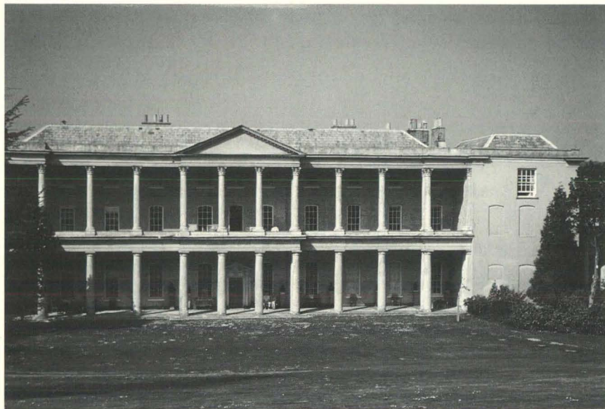
Fig. 2. West Wycombe (Buckinghamshire): façade sud.
